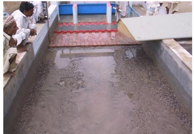
Fig 4a existing condition (stone displaced)
