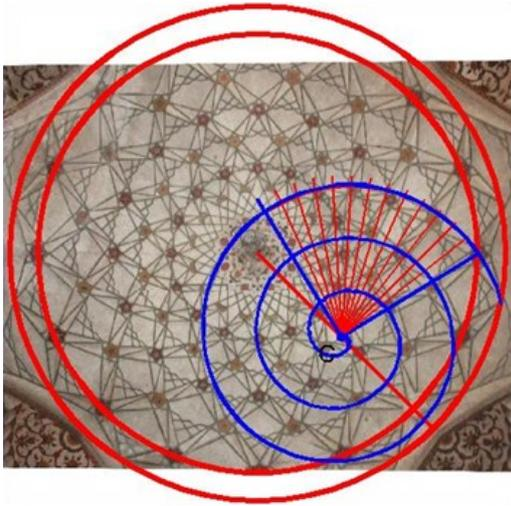
**Fig. 15:** Logarithmic spiral superimposed on the dome
