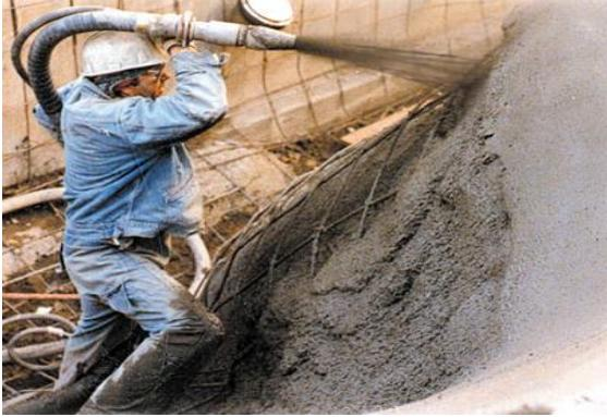
**Fig. 2:** Shotcrete or spraying concrete (proshot concrete PC)
