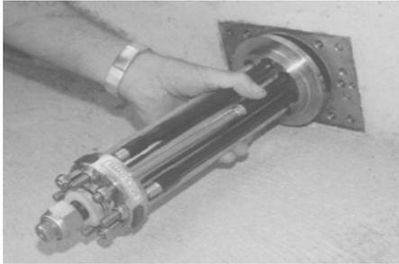
**Fig. 16a:** Fe-SMA device at Basilica San Francesco at Assisi Italy, for earthquake protection (Janke, 2005)
